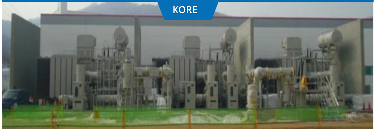
154KV 125MVA LS Electric Paju
