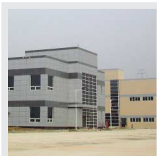
Wuxi Plant (China)
